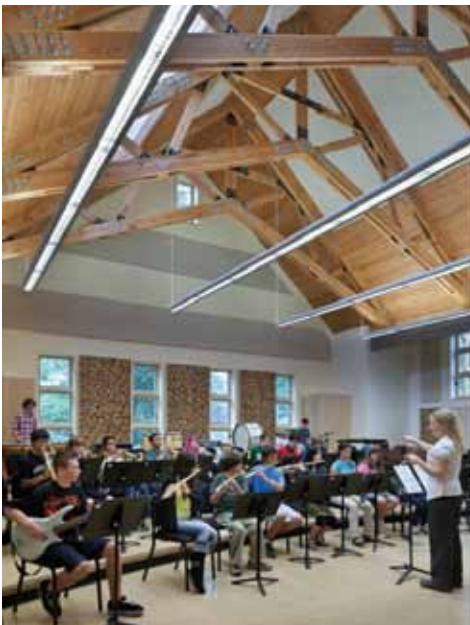
The Music and Science Building replaced a 1940s bus storage barn previously located at the site. This structure was carefully deconstructed, and the new building's wood scissor trusses were created from the materials set aside.
