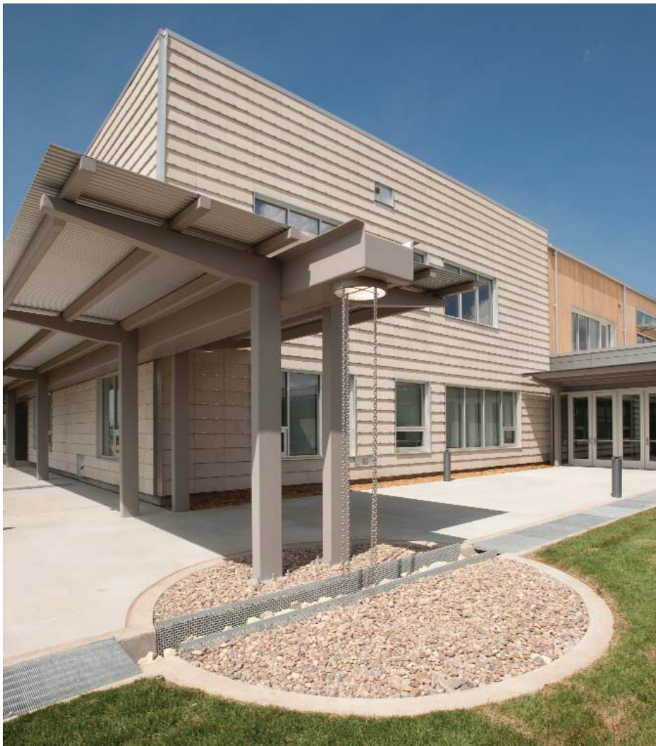
Front entry to the Kiowa County School. Evident in the picture is water recovery/storage, native limestone cladding and reclaimed cypress.
