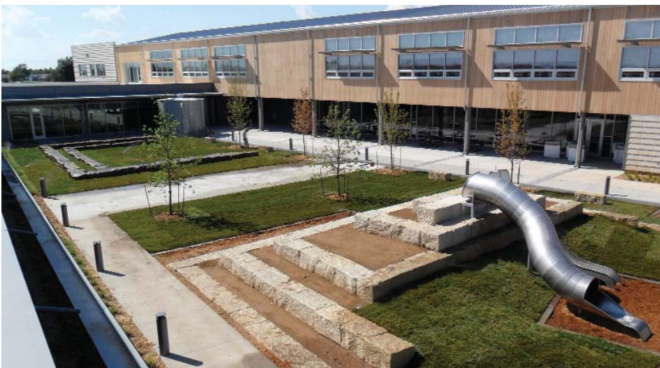
Courtyard area illustrating the light shelves on the second story classrooms and one of the six water cisterns which store 121,000 gallons of water for irrigation.
