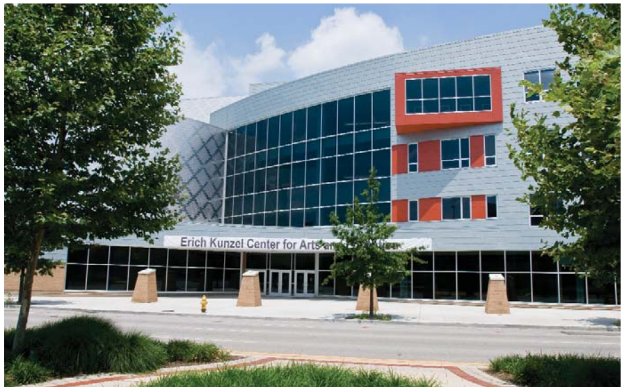
The primary southern entrance with its volume enclosed with curtainwall, the zinc metal panels proceeding from the east side leading over the entrance glazing producing the building signage backdrop.
