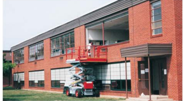
DURING... installation can even take place with classes in session. Factory pre-assembled.
